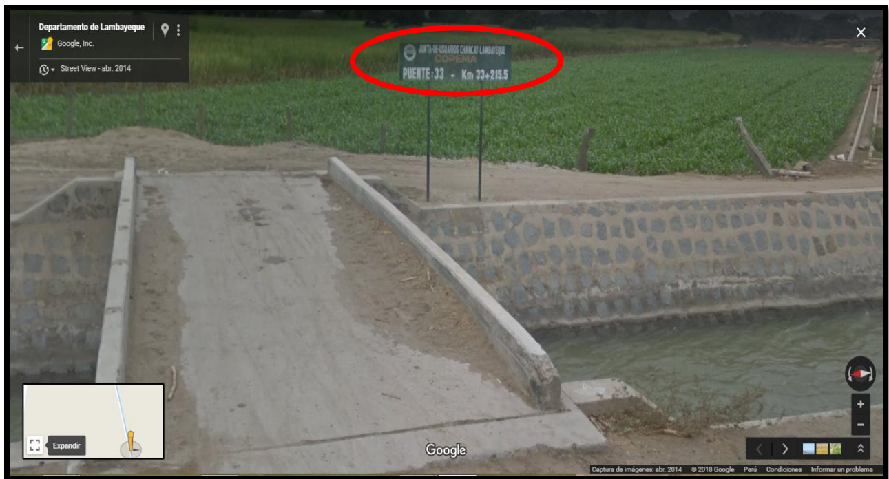
Figura 66: Canal Taymi, Km 33+215.5, fuente (google maps)
