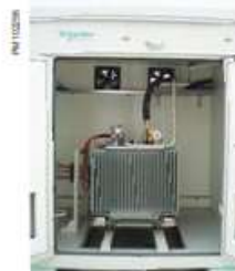
Transformer in PV box
