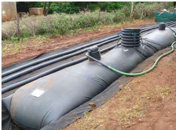
Figura 11: Biodigestor tubular
