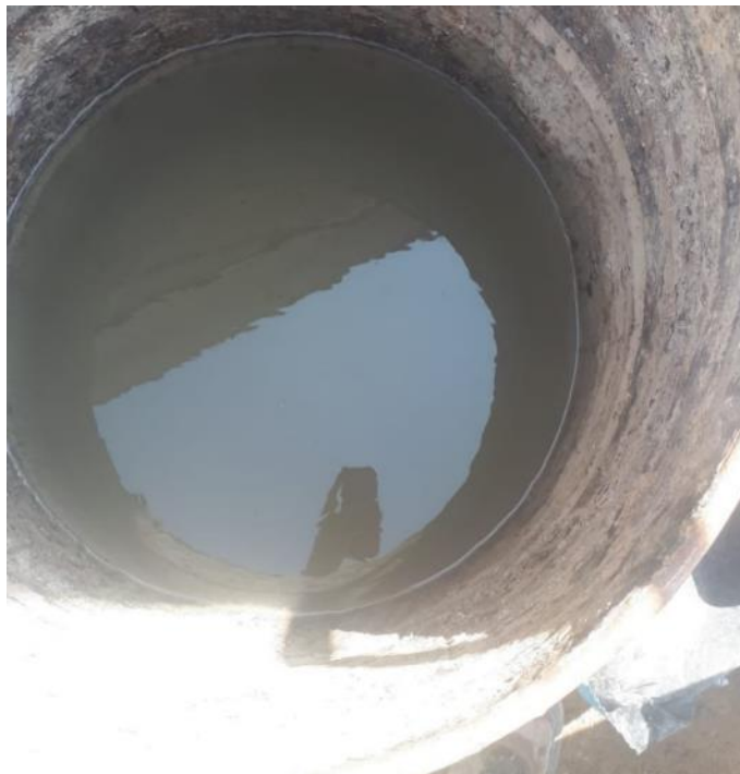
Fig. 71. Agua Potable – Laboratorio “LEMS W&C EIRL”
