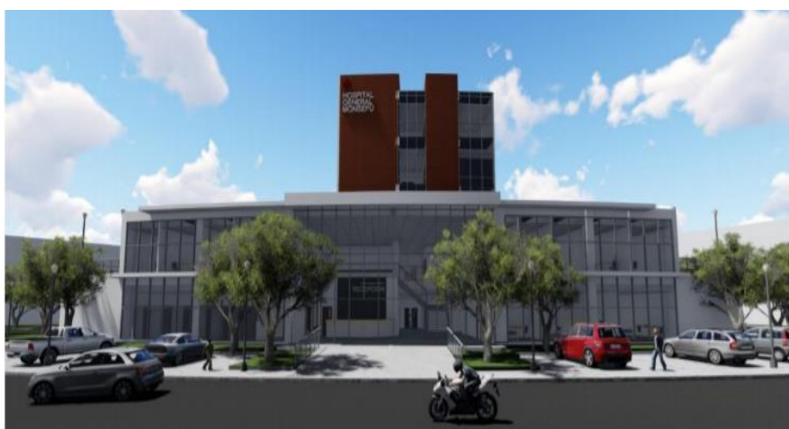
Figura n° 6. Hospital General de Monsefú.
